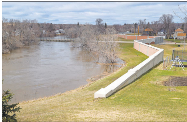
The floodwall near Riverview Drive is seen in Valley City on Monday.
