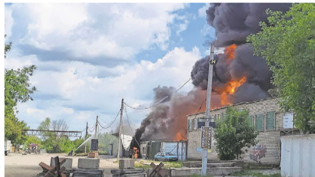
A structure on fire in May 2022 after a bombardment in Pavolgrad, Ukraine, about 10 miles from the front lines.
