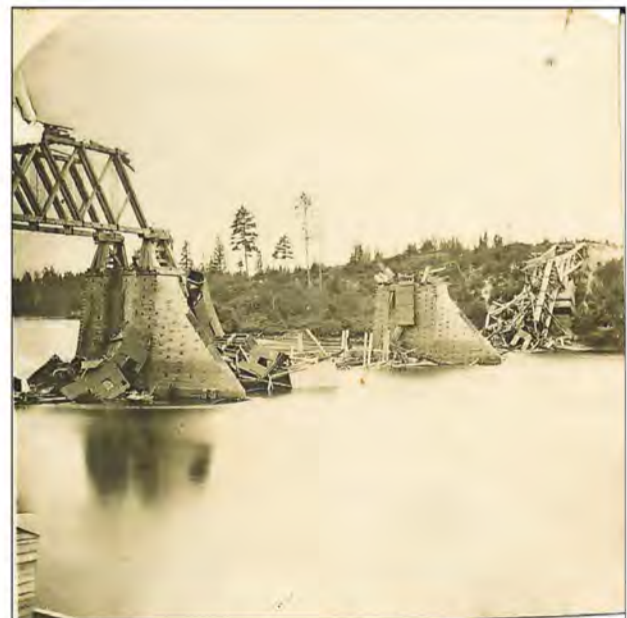
Contributed / Crow Wing County Historical Society Museum Built in 1871, the Northern Pacific Railroad bridge across the Mississippi River in Brainerd collapsed under the weight of a train on July 27, 1875.
