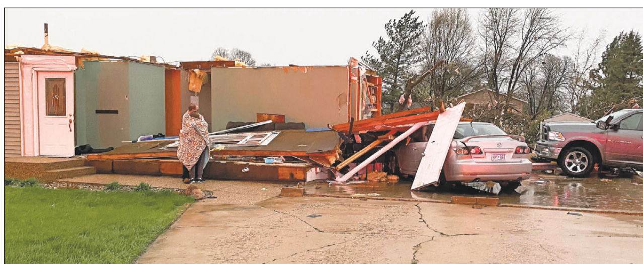
The owners of a home on the corner of West Meadow Lane and Donna Drive in northwest Alexandria look at what's left of their home after a storm whipped through the area Thursday.
