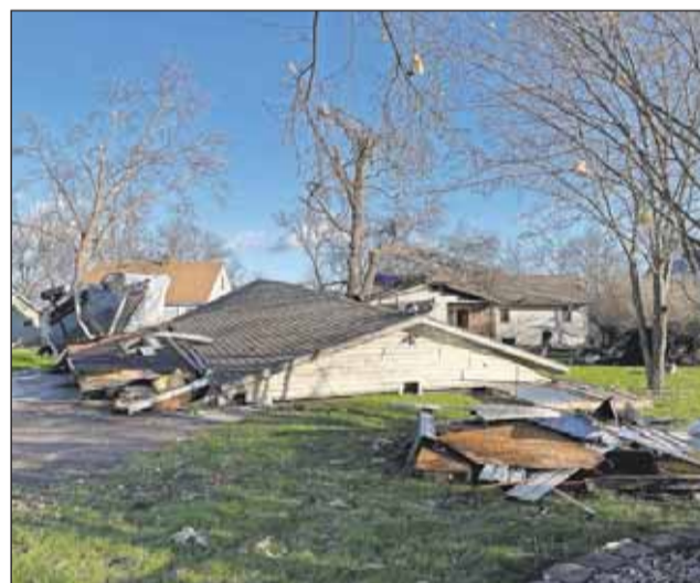
A boat overturned, a garage collapsed and trees went through a house on South Lake Darling Drive owned by Chad and Heidi Schroeder. A storm hit Douglas County shortly after 7 p.m. Thursday. Many areas around the county were hit hard and damage is widespread.
