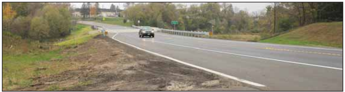
The bridge over State highway 87 is officially open to the public. Those traveling on the newly constructed highway may also notice the widened shoulders.
