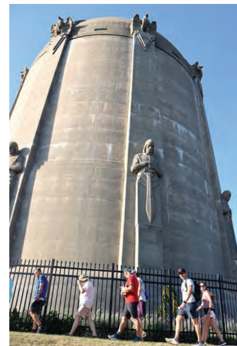
The Washburn Park water tower was designed by Henry Wild Jones, a neighborhood resident. (Photo by Tesha M. Christensen)
