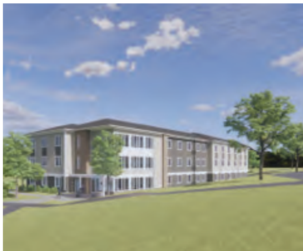
Pictured is a rendition of the new residence hall being built on the Crown College campus. (Submitted photo)
