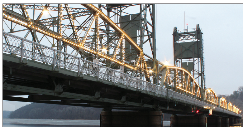
Last year the city installed lights on the south side of the historic lift bridge, this year the city will pay for installation on the north side and rely on downtown businesses to fund installation for the south side. (Gazette file photo by Matt DeBow)
