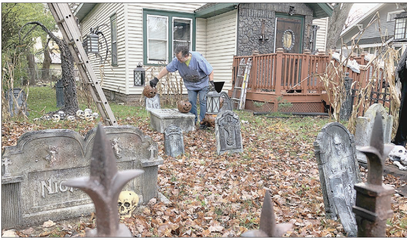
Bill Nicholson works in the front yard of his home at 330 Fourth St. in Cloquet Tuesday morning, placing a quartet of fanciful pumpkins just so and wrapping up construction of a new mausoleum that will house a fog machine on Halloween night. Nicholson is preparing for the big show on Sunday, which should start at his house after 4:30 p.m.
