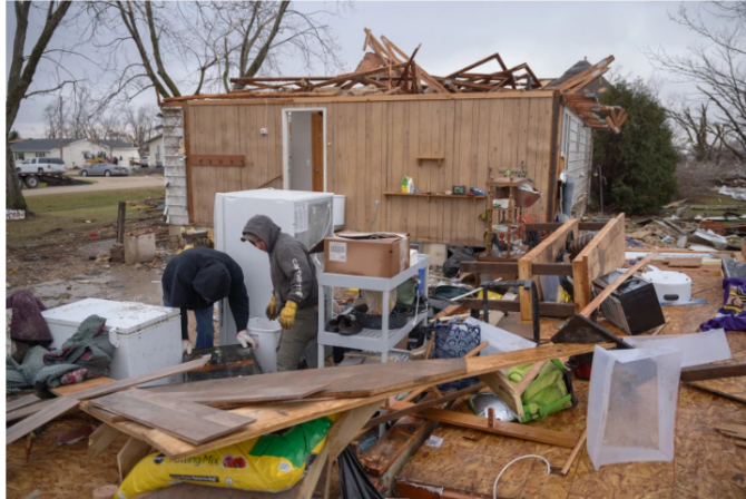
Matt Carpenter, left, and friend, Ryan Hanson, help clean up debris in what used to be the garage of Carpenter's father-in-law, Terry Voigt, on Wednesday, April 13, 2022, after a tornado the night before in Taopi, Minnesota. The National Weather Service confirmed an EF2 tornado touched down in Taopi. Joe Ahlquist / Post Bulletin
