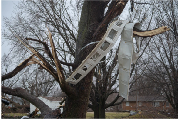
Damage to structures, trees and vehicles on Wednesday, April 13, 2022, in Taopi, Minnesota. The National Weather Service confirmed an EF2 tornado touched down in Taopi. Joe Ahlquist / Post Bulletin
