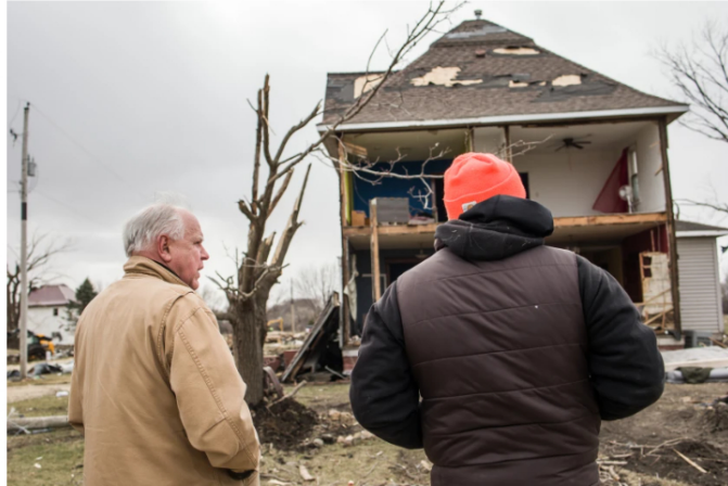
Gov. Walz surveys tornado damage on Thursday, April 14, 2022, in Taopi, Minnesota. The National Weather Service confirmed an EF2 tornado touched down on Tuesday evening, April 12, 2022. Traci Westcott / Post Bulletin
