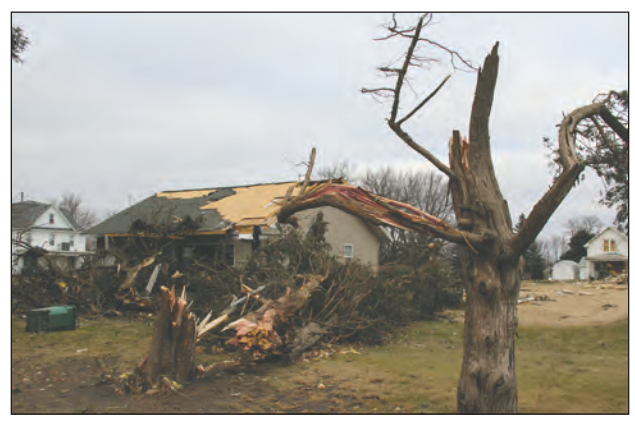
Several homes sustained major roof damage during the storm. SARAH STULTZ/ALBERT LEA TRIBUNE
