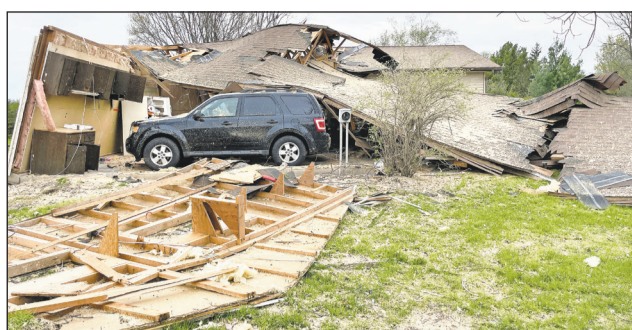
Photos by Celeste Edenloff / Alexandria Echo Press Dustin and Desiree Wiita of Alexandria, lost not only both their vehicles that were parked in their garage, but most of their house when a tornado ripped through their neighborhood along South Darling Drive on May 12.
