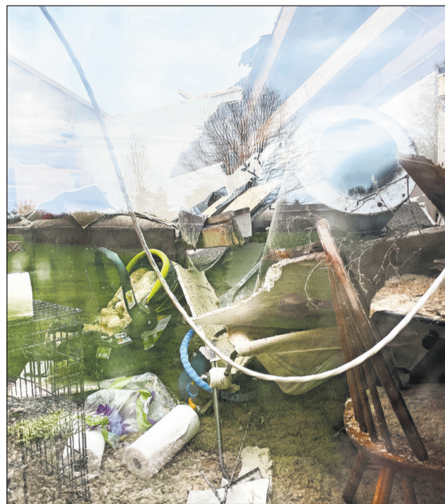
Looking through a window of a home owned by Dustin and Desiree Wiita of Alexandria, a car seat for their baby can be seen. The seat is sitting among all the debris and pieces of their roof after a tornado ravaged their home on May 12.
