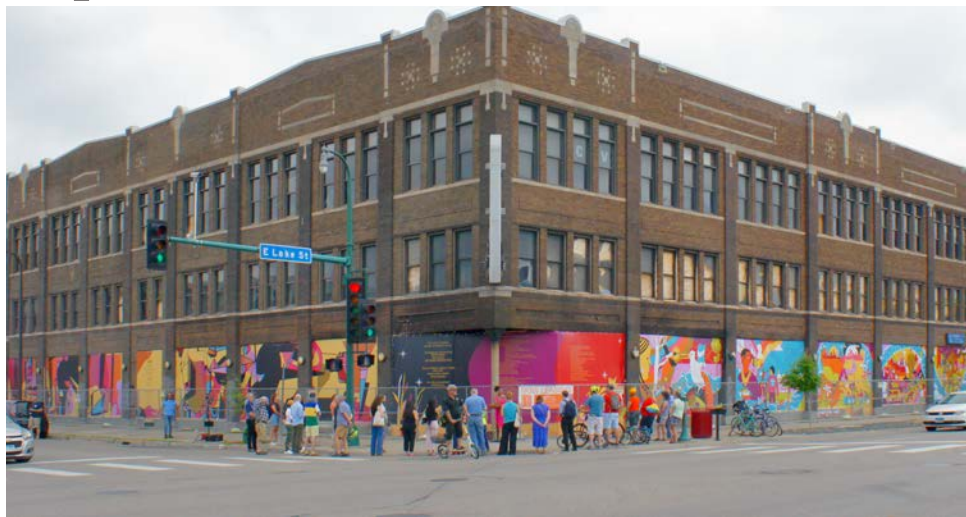
A series of poems and colorful murals are displayed on the first floor of the Coliseum building. At right, Tish Jones of TruArtSpeaks talks about the project on July 11. The building renovation project is $2 million shy of the funding needed to start. (Photos by Terry Faust)
