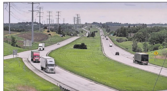
Courtesy of the Minnesota Department of Transportation Cars and trucks rumble over Interstate 94 east of Fergus Falls, Minn., on Thursday, May 27.
