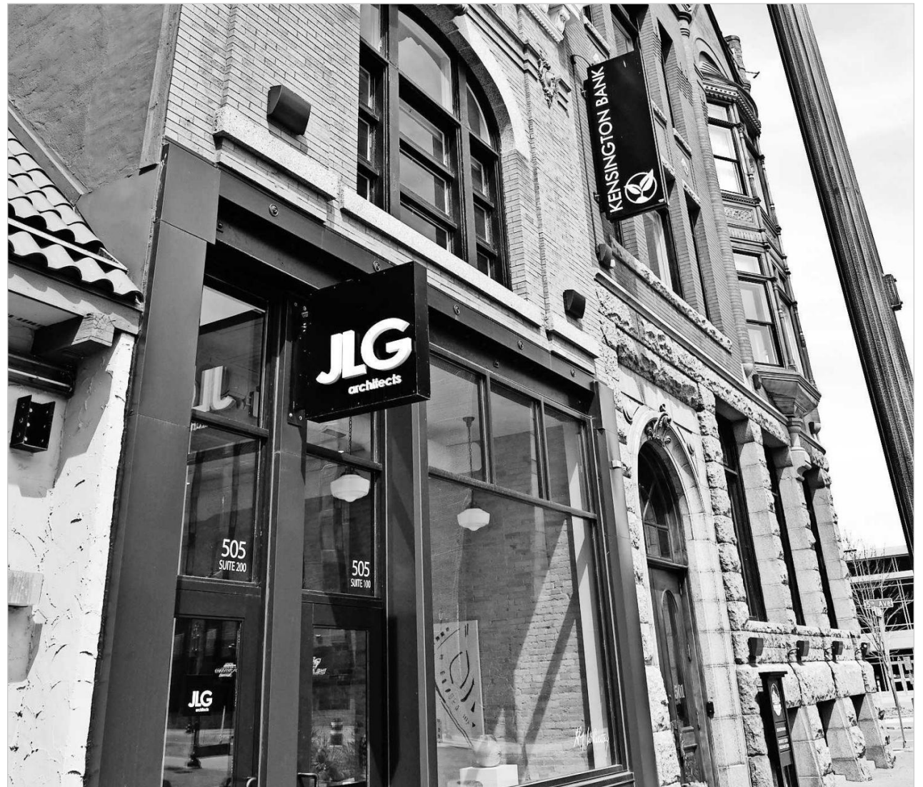
The recently renovated Whitney Building is pictured Friday, April 16, 2021, in St. Cloud. DAVE SCHWARZ/DSCHEWARZ@STCLOUDTIMES.COM
