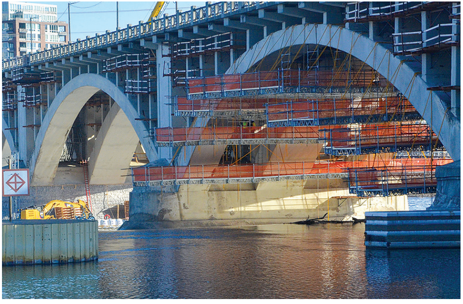
Top: South side of Third Avenue Bridge, with railing removed. Bottom: North side, with scaffolding, over the falls. After the lower structural repairs are complete, the bridge deck will be rebuilt.
