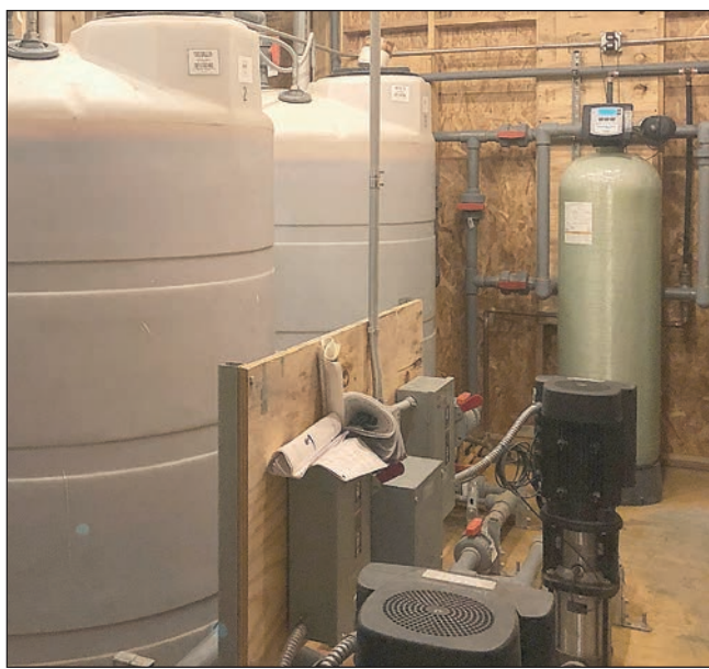
The Kwik Trip store on Minnesota Highway 210 has two wells which provide water the store must filter for sediment. Additionally, because of the low supply of water, Kwik Trip installed three 1,000-gallon tanks to store enough water to make sure the store has enough water to flush all the toilets and supply other water needs at any given time. A layer of reddish dust — dried sediment — coats the floor and pipes around the tanks. The poor quality of the water is also hard on the machines in the store. Jana Peterson / Pine Knot News
