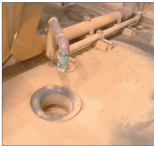
The Kwik Trip store on Minnesota Highway 210 has two wells which provide water the store must filter for sediment. Additionally, because of the low supply of water, Kwik Trip installed three 1,000-gallon tanks to store enough water to make sure the store has enough water to flush all the toilets and supply other water needs at any given time. A layer of reddish dust — dried sediment — coats the floor and pipes around the tanks. The poor quality of the water is also hard on the machines in the store. Jana Peterson / Pine Knot News
