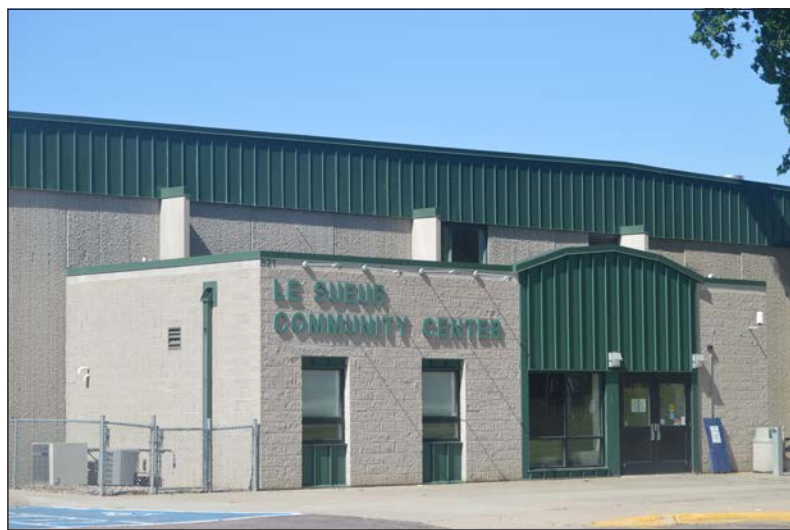
The Le Sueur Community Center will be closed for the rest of the year if no stimulus funds are available to the facility. The city council made the decision after finding that they could not open the Community Center without a significant budget deficit. (Carson Hughes/Le Sueur County News)
