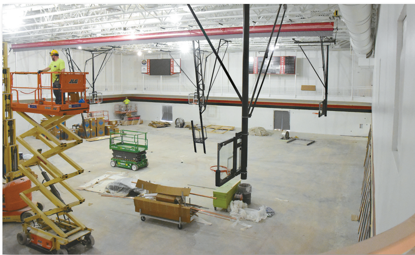
Painting begins before the floor is laid to prevent any damage to the floors.
