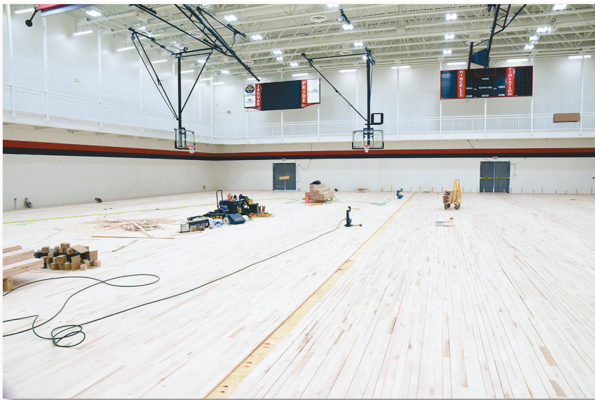
Basketball floor construction began on Wednesday, May 1. The floor consists of three layers. Layer number one is sleepers, two by three-inch strips of wood, which are spaced and nailed to the cement. This provides a solid base for the maple flooring. Next comes the plywood, nailed to the strips of wood. Finally, the grade A2 maple flooring is nailed to the sub floor at a right angle to the sleepers and plywood. Every four feet, there is a 1/16 of an inch space left for expansion and contraction of the wood. Through the entire perimeter of the floor, there is a two-inch space left for the same reason.
