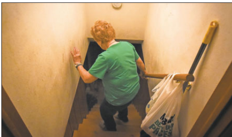
Jillian Gandsey | Bemidji Pioneer Janet Dreyer walk down the stairs into her basement on Wednesday where a water main break caused a sewage backup in May.
