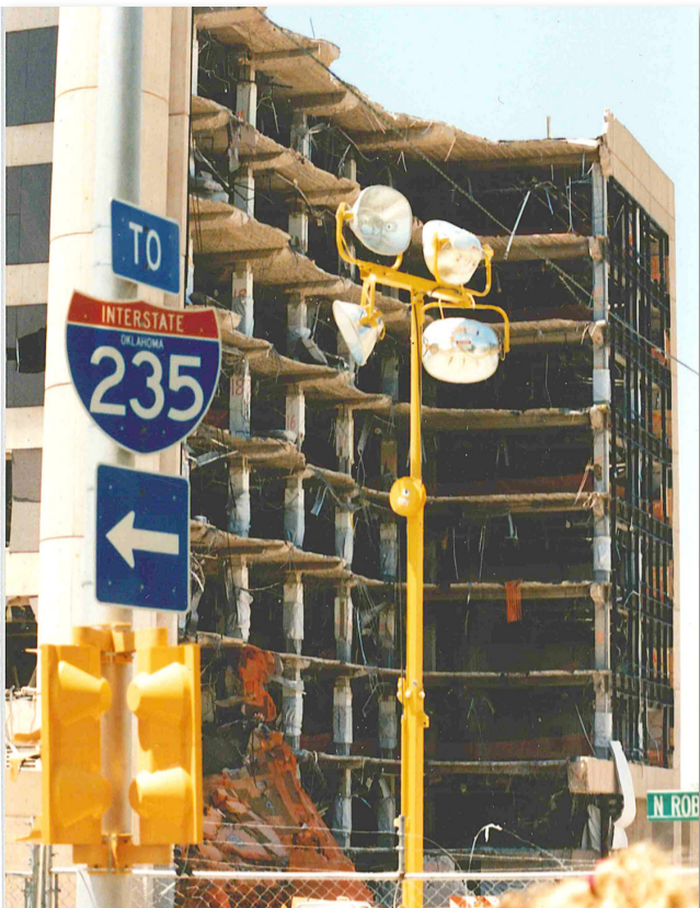
The damage done to the north side of the Murrah Building after the bomb. This photo was taken just before they imploded the building.
