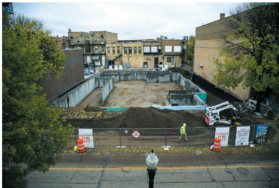
Construction continues on a building on the former Arbor Park site in downtown Grand Forks.
