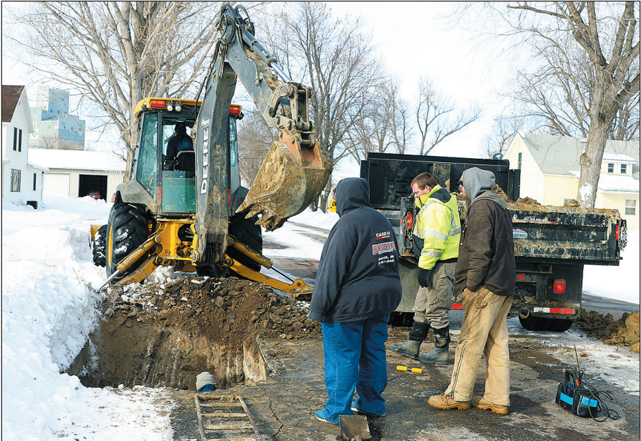
Ellsworth Mayor Tasha Domeyer, center, looks on Wednesday afternoon as Orv's Plumbing & Heating digs an exploratory hole in search of a leak in the water main on Maple Street. Tim Middagh / The Globe
