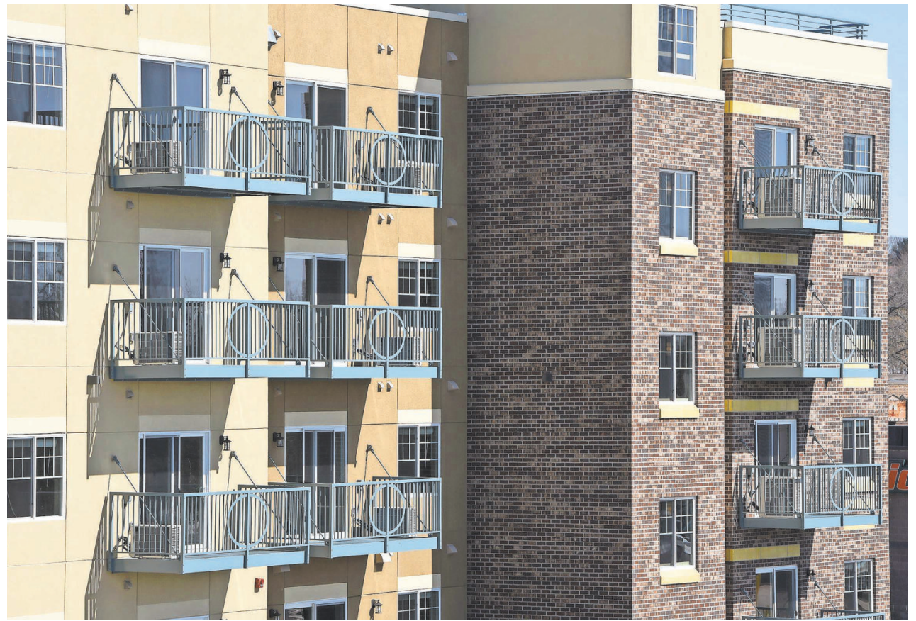
The new Mississippi Lofts apartments are pictured Thursday, March 29, in Sauk Rapids. The complex opens Friday. About 40 of the 57 apartments have been rented already. DAVE SCHWARZ, DSCHWARZ@STCLOUDTIMES.COM
