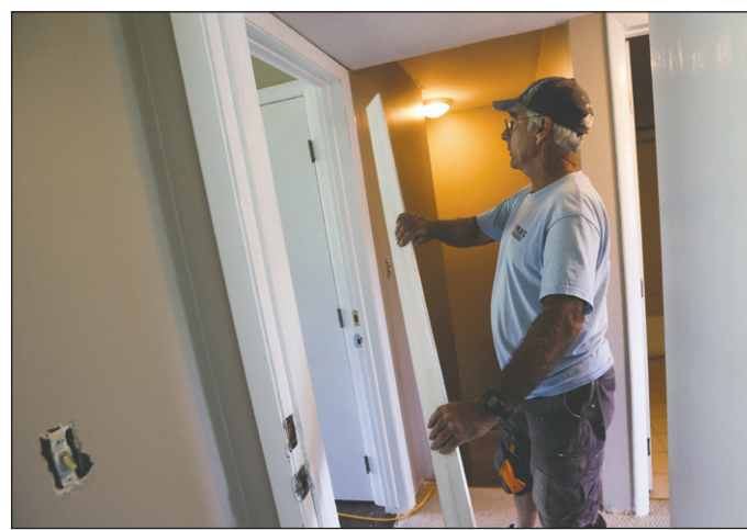
Volunteer K.C. Reed on Wednesday installs baseboards in an apartment at Bear Creek Church Housing in Rochester.
