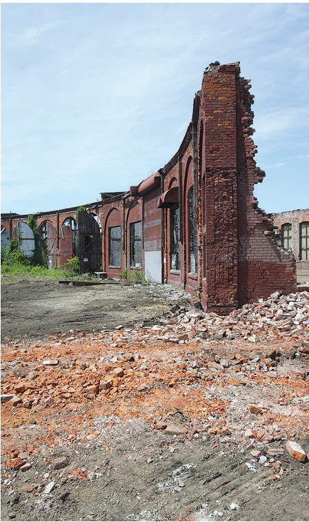
Shoreham roundhouse, July 31, 2019. (Photo courtesy of Charlene Roise)
