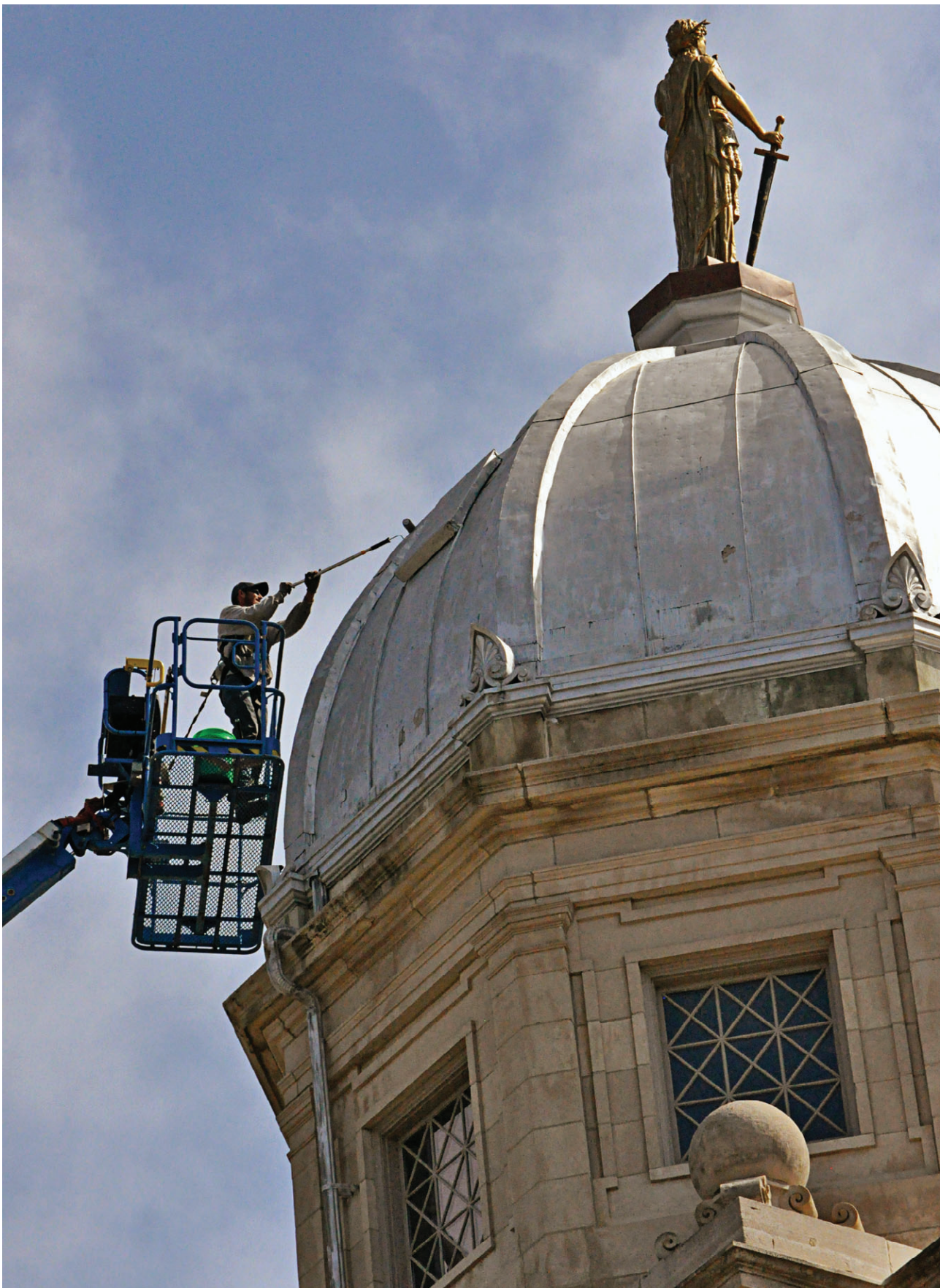
Adam Sandmeyer of Mankato-based Schwickert's Tecta America works to seal and repaint the leaky dome of the historic Jackson County Courthouse Tuesday morning.
