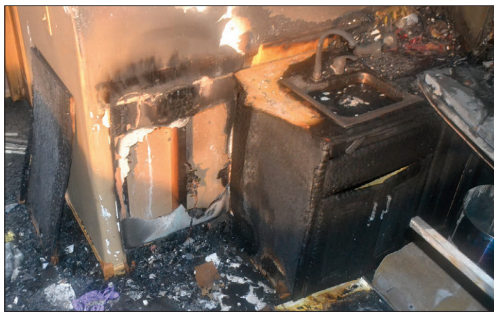
A fire that apparently started with small refrigerator caused significant damage to the basement of the home at 1257 129th Lane in Coon Rapids April 10. Photo courtesy of the Coon Rapids FD
